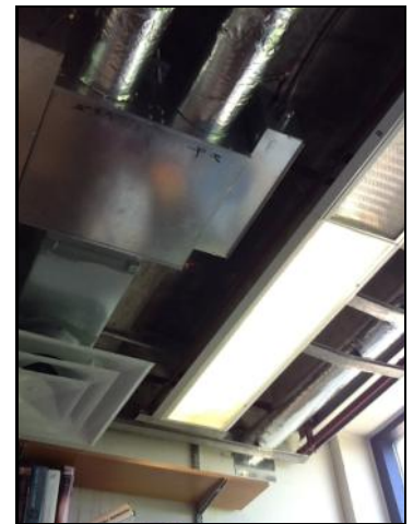
Open ceiling in a faculty office. Parker building - June 5, 2012
