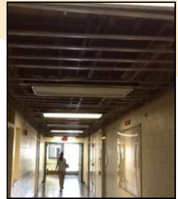
Wide open ceilings above a hallway in the Parker building. June 5, 2012
